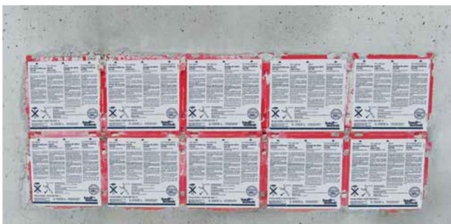
double wall insert HSI150 as block assembly
