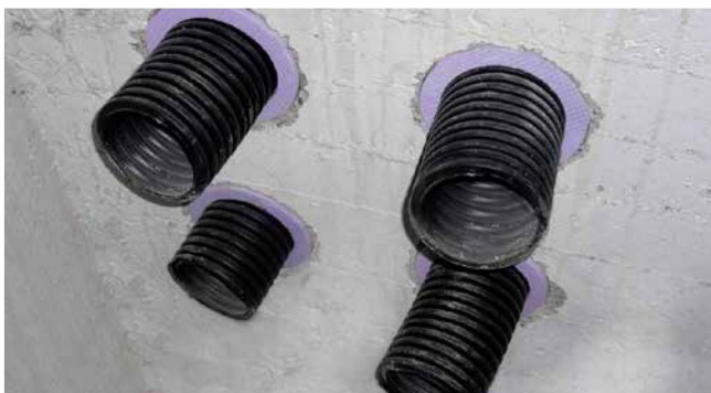
view of inside of building (insulation ring)
