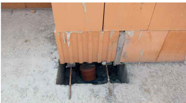
difficulty: retrofit gas-tight and vapour-proof sealing
