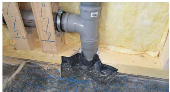
difficulty: integration of vapour barrier foil
